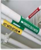
Colour coding of water piper to avoid contamination
